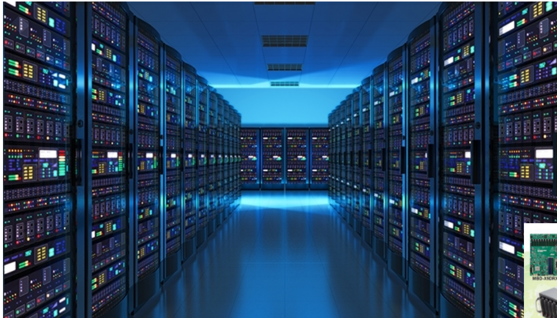
Cited source : https://globemoving.net/blog/moving-fully-populated-server-racks-during-data-center-relocation/
